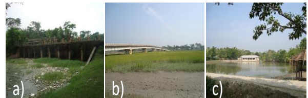
Fig. 4 a) Water logging due to construction of sluice gate at Foila Bazar; b) bridge on the Daudkhali river course which enhance sedimentation in the river bed at Talbunia, Rampal, Bagherhat; c) playground of Talbunia primary school, Talbunia, Rampal, Bagherhat becomes a permanent water body.
