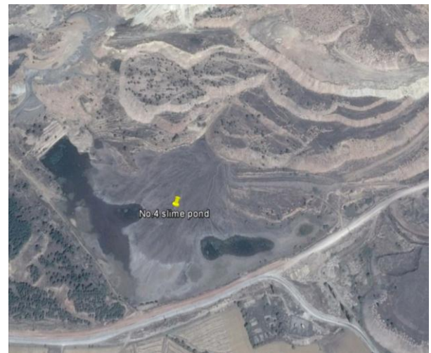
Fig. 5 Slurry pond formed in the hole of No 4 mined out pit.
