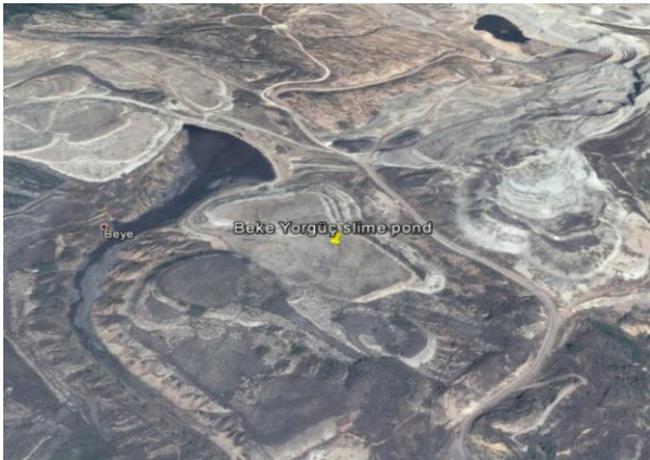
Fig. 6 Slurry pond formed in the mined out hole of Beke open pit.
