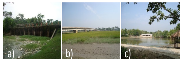
Fig. 4 a) Water logging due to construction of sluice gate at Foila Bazar; b) bridge on the Daudkhali river course which enhance sedimentation in the river bed at Talbunia, Rampal, Bagherhat; c) playground of Talbunia primary school, Talbunia, Rampal, Bagherhat becomes a permanent water body.
