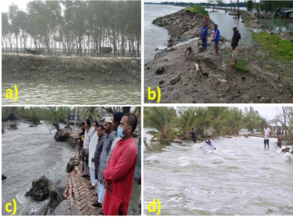
Fig. 6 a) Weak embankment at the right bank of the Kabodak river at Pratapnagar, Asasuni, Satkhira; b) The collapsed embankment of 35/1 polder of Water Development Board (WDB) in Sharankhola upazila of Bagerhat by Cyclone Amphan (Anon, 2020d); c) A broken road submerged in water due to cyclone Amphan (Islam, 2020a); d) Saline water overtopped the river banks due to cyclone Amphan (Islam, 2020b).
