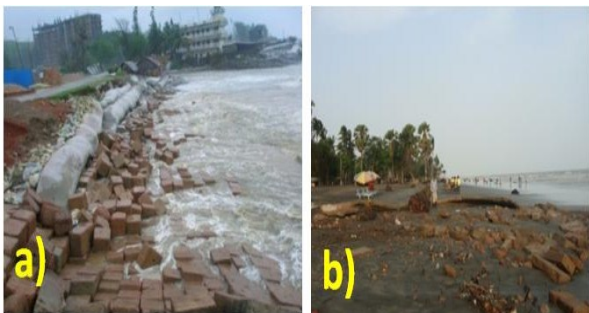
Fig. 5a) Severe erosion occurs at Kalatoli beach, Cox's Bazar due to cyclone Mahasen; b) Severe erosion occurs at Kuakata beach, Kalapara, Patuakhali due to cyclone Mahasen.
