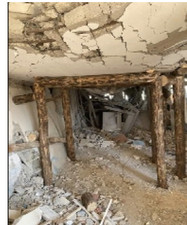
Fig. 7 Supporting work for roof and side walls control.
