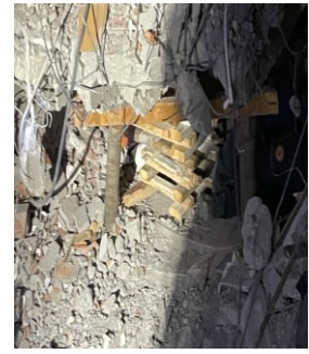
Fig. 8 Wood crib reinforced supporting work.
