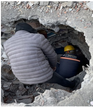
Fig. 5 Shaft-shaped search and rescue operation.
